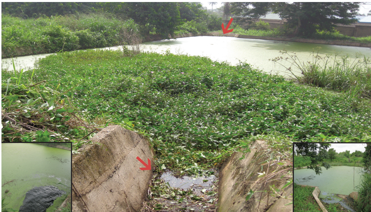
FIG. 1. The leachate pond - arrows show the inlet and outlet channels; inset, below left, is the leachate surface covered by floating macrophytes while inset, below right, is the outlet channel.
